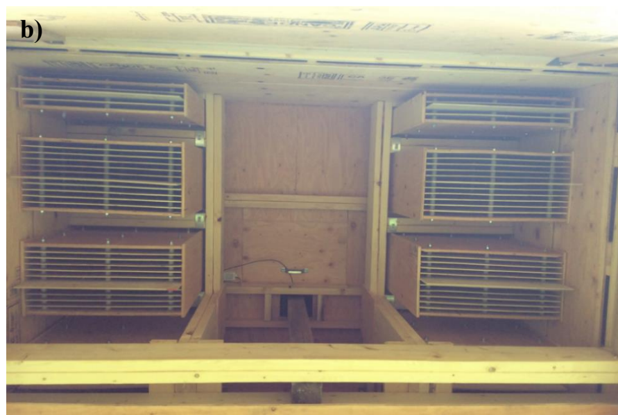
Figure B.3. Exterior (a) view of the unoccupied (as of 2021) mini-condo, Condo C and (b) interior view, looking up at half of the baffled roost boxes within the Condo C in the Kootenay region of British Columbia, Canada. (Photos: S. Dulc)
