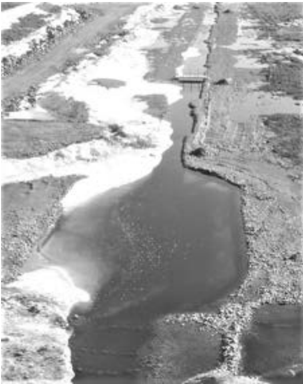
Figure 2-26 Looking upstream to large pond and bridge location of Camera #1 and #2 installation (photo credit: ERM)
